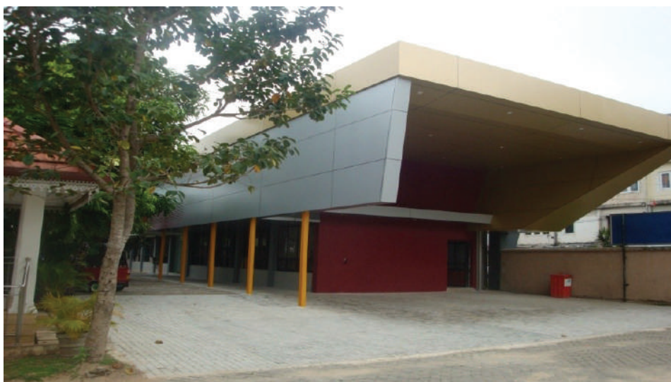
G.P.S. Control Room
