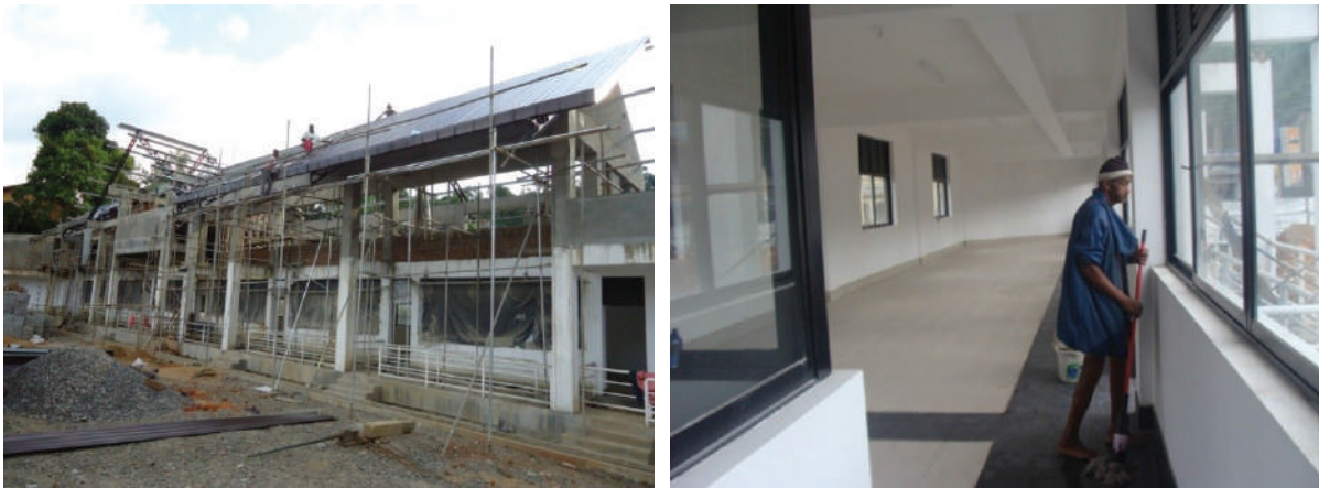
Talawakalle Bus Terminal Site under construction
